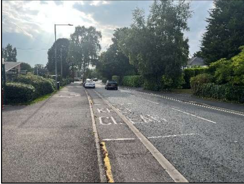
Figure 9: Hagley Primary School
