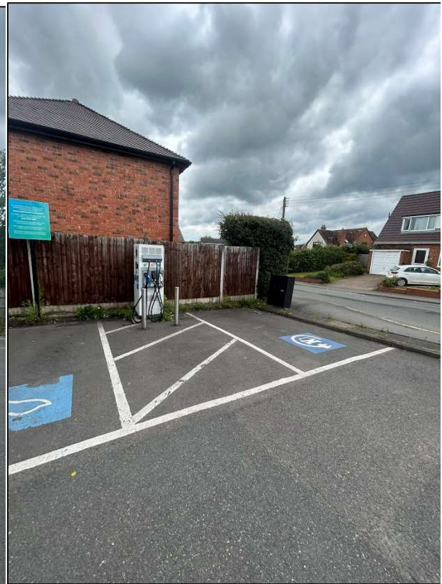
Photograph 11: Catshill Car park
